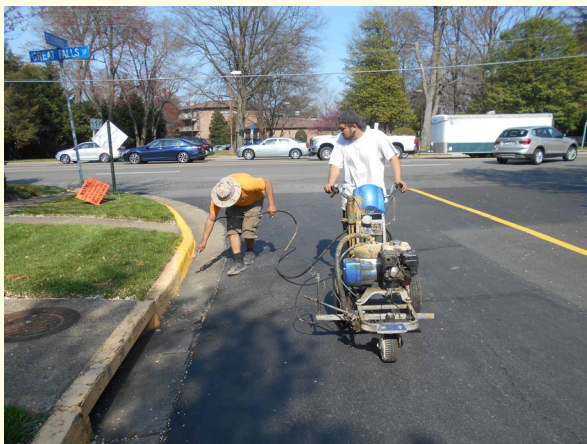
Our yellow curbs were re-painted by our streets contractor
